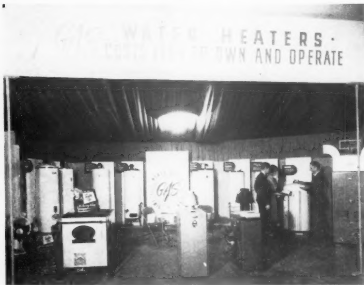
Display of automatic water heaters and appliances. From left to right the water heaters are Ruud, Mission, Day & Night, Crane, Rheem, General, Continental and Servel. In the foreground are a Ward floor furnace, a Bryant boiler and a Crane boiler. A Coraire warm air furnace is at the extreme right.
